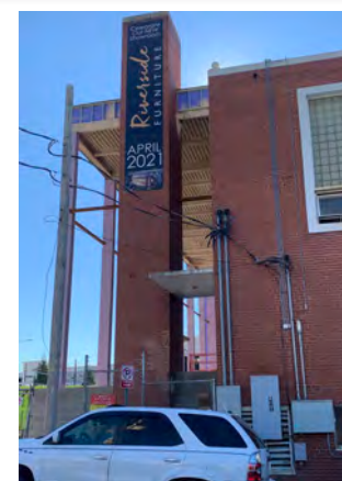
Construction is underway near the Textile Tower on Main Street.
